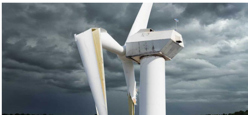
Figure 1: Damaged Wind Turbine Blade. Source: https://www.windturbinemagazine.com/why-do-wind-turbine-blades-wear-out/ .
